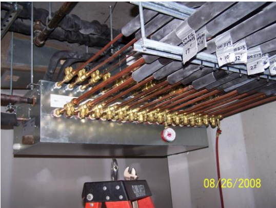
The picture above depicts a BC Controller that connects the refrigerant piping from the 16 individual room units to the outdoor unit.
