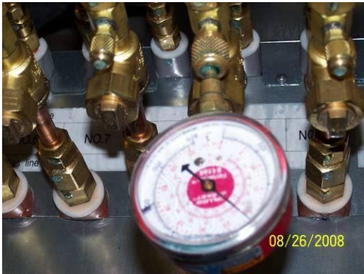
The picture above depicts a BC Controller that connects the refrigerant piping from the 16 individual room units to the outdoor unit.
